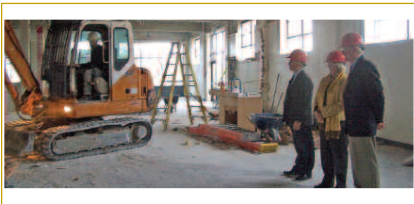
Ada County Commissioners at facility during remodeling.
